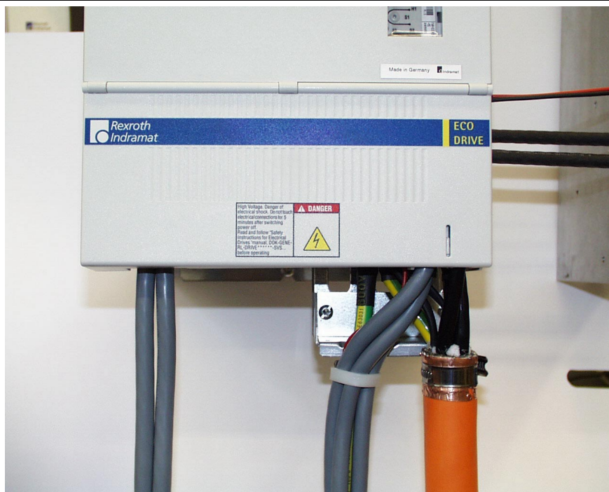
Fig. 16-32: View with contact protection
